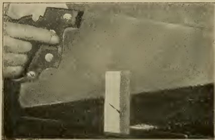
Fig. 191—Ripping Triangular Glue Blocks
